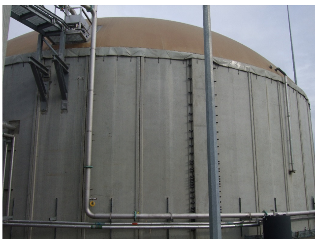
Figure 4.1: Pre-cast sectional concrete tank
