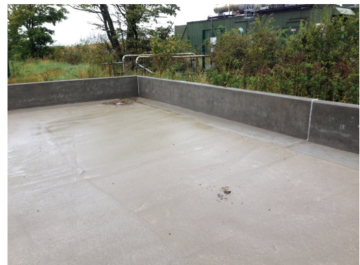
Figure 4.6: Example of a bund wall and sealed surface
