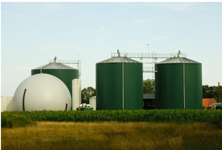
Figure 5.2: Spherical floor-mounted dual membrane 'gas bubble'
