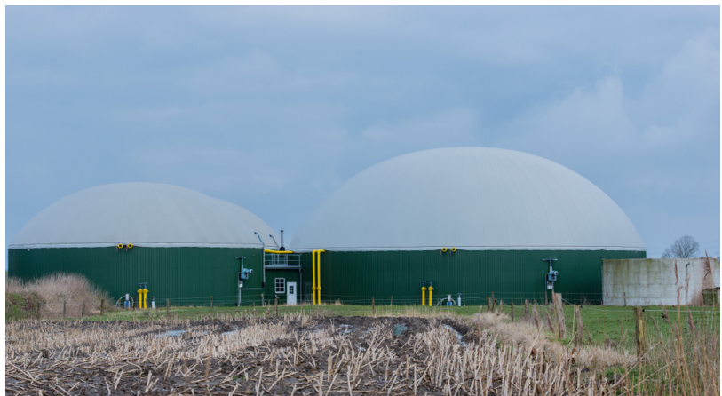
Figure 5.1: Flexible dual membrane on top of tanks
