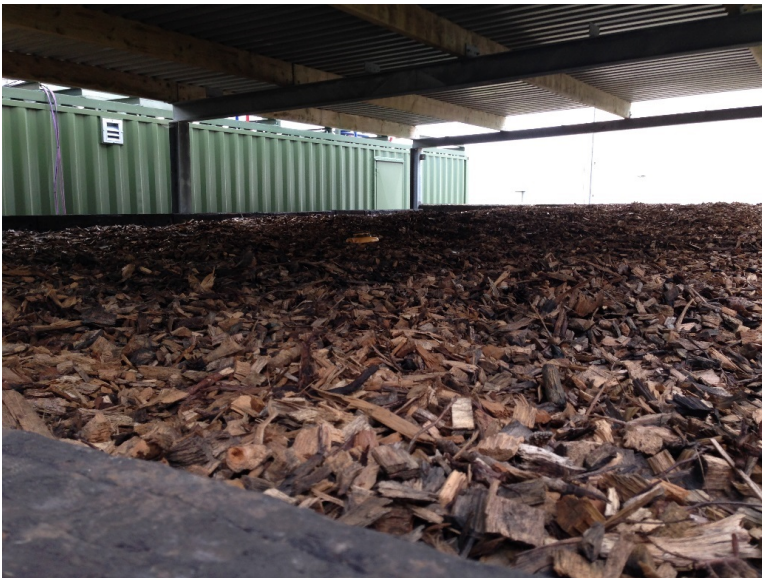
Figure 7.1: Open woodchip biofilter
