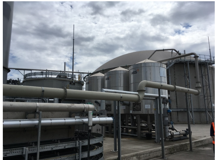
Figure 4.5: Example of a three-tank pasteurisation system
