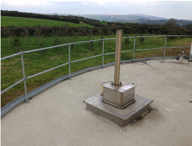
Figure 4.2: Example of water-based pressure relief valve
