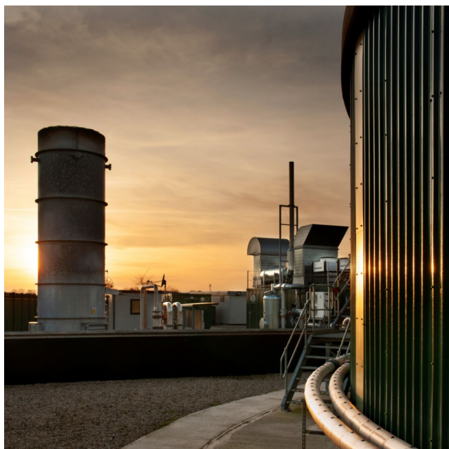
Figure 5.4: Enclosed flare at an AD facility 10
